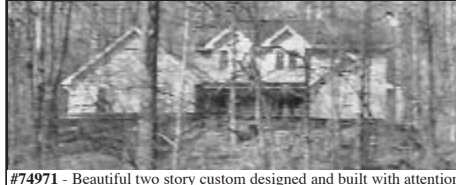
#74971 - Beautiful two story custom designed and built with attention to detail. Hardwood floors throughout with beautifully finished staircase and many special touches. Very secluded, but close to I-79. Enclosed play area in back. 12x32 workshop with electricity. Great deck in back. 6 acres, mostly wooded. Stream on property. $299,000. Call Doris for appt. 304-672-4545
