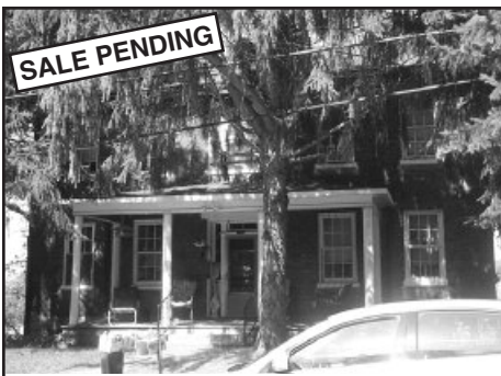
GERMAN TWP. - All brick two story farm house with outbuildings on over 7 acres!
